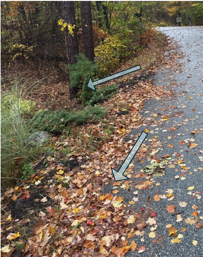
Roadside ditch erosion with some gullies draining into private property (left) and others directing flow into a catch basin that discharges directly to the lake.
