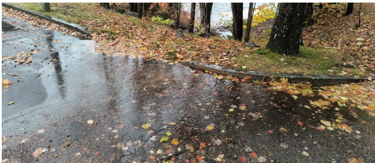
Looking up Coot Bay Drive, where runoff (with high road salt concentrations in winter) flows down the road surface (top left). Water pools in a low point in the road (bottom) before flowing to the lake through a small, steep wooded area with limited ground cover and minimal pollutant attenuation (bottom and top right).
